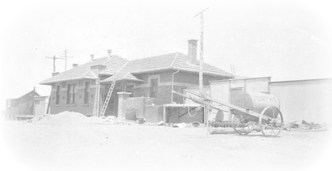
Balranald Telegraph Station Building
