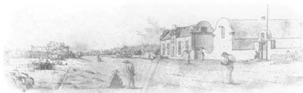
View of Church Street in Graaf Reinert
